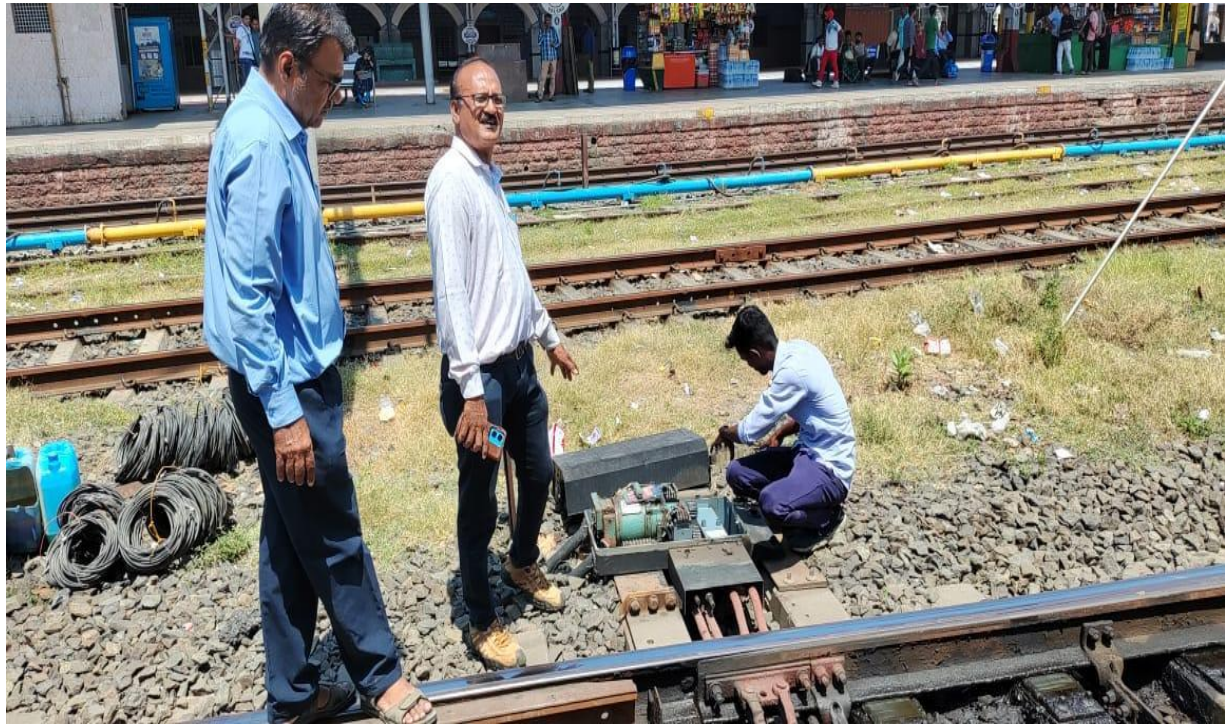
Site Visit: Railway Station, Valsad 03/05/2023
